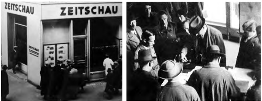
Figure 3.4, 3.5: Zeitschau Storefront, Outside and Inside, Am Tuchlaubenplatz, 1 st District, Vienna
