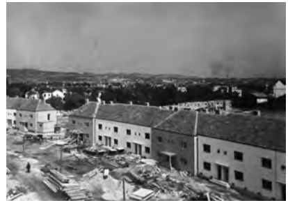
Figure 1.3: Settlement under Construction
