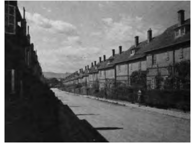
Figure 1.8: "Hoffingergasse," Architect: Josef Frank
